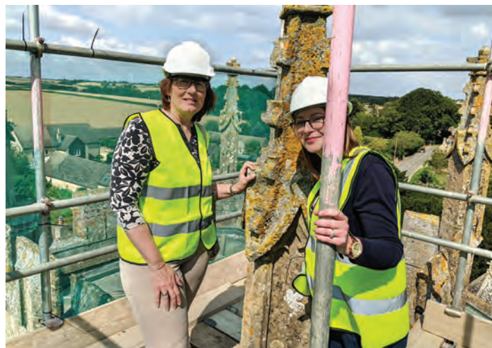
Jennie Schillig (left) and Sophie Hammond inspecting stonework repairs to the tower at Chadlington.
