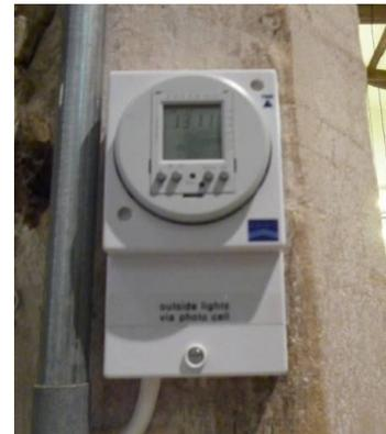
Figure 2. External lighting controller
