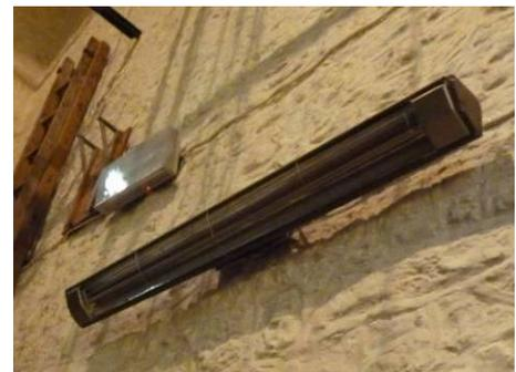
Figure 5: Radiant heater
