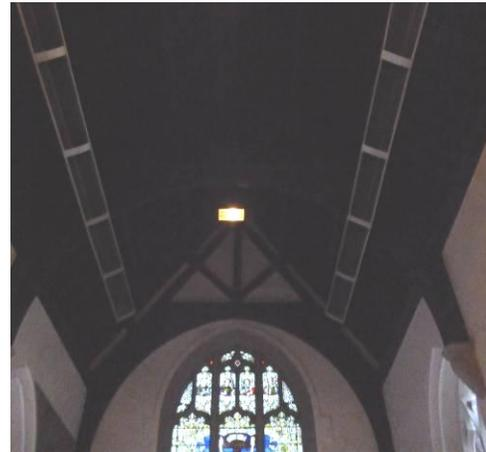
Figure 3. Radiant heaters
