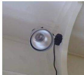
Figure 1. Reflector spot lamp
