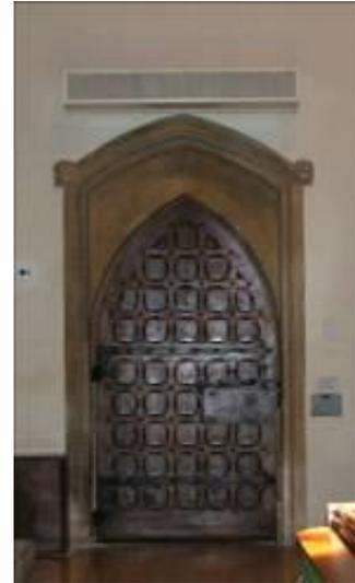
**Figure 5: Example of an air curtain in a church**
