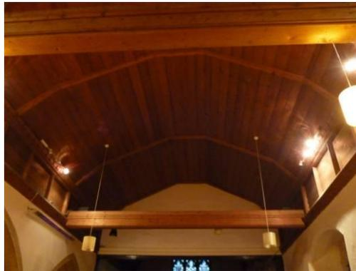
Figure 4. Barrelled main aisle ceiling
