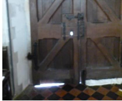
**Figure 6. Gap under south aisle door**
