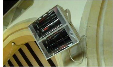
Figure 5. Radiant heater
