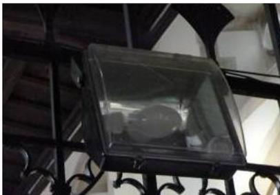
Figure 1. High pressure sodium lamp in Chancel
