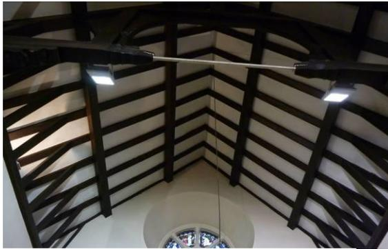
Figure 3. Halogen linear lamps
