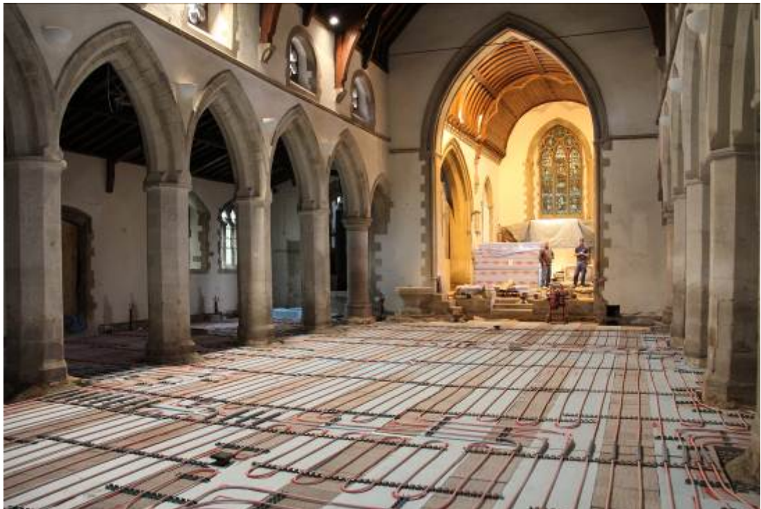
Above: under-floor heating being installed
