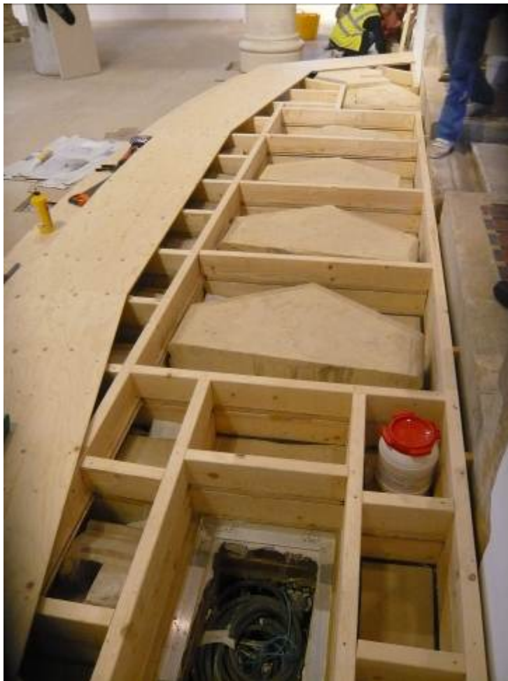
Above: Construction of the dais underway
