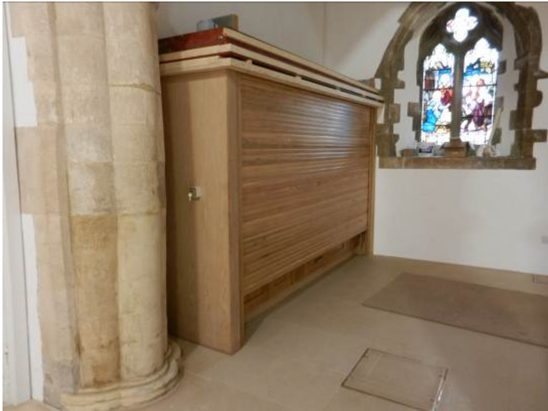
Above: The new servery with roller-shutter
