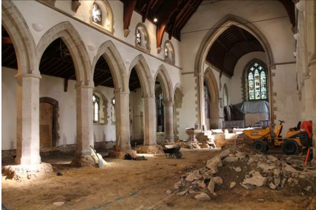
Above: the excavation of the nave
