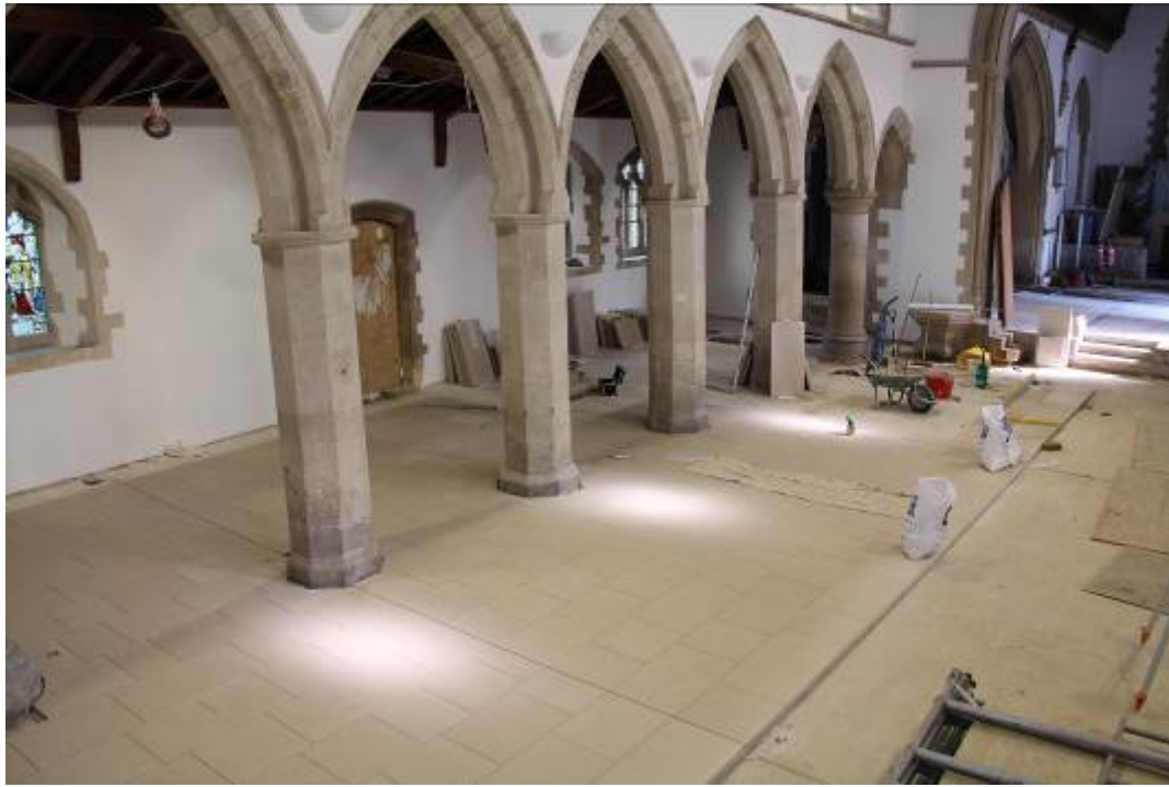
Above: Laying the paving slabs in the nave
