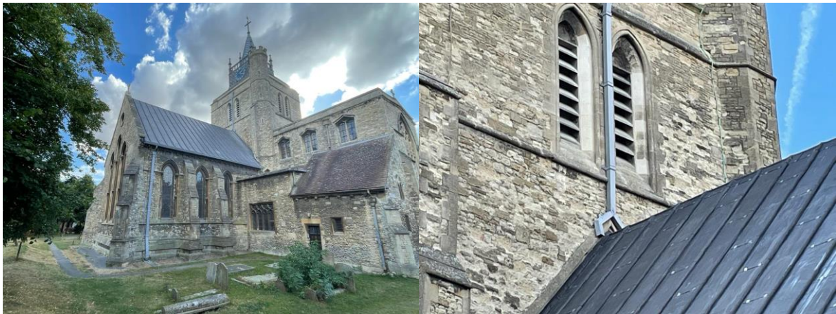
Aylesbury, St Mary – completed repair of chancel roof and tower stonework
