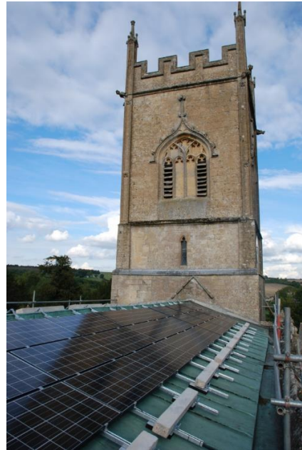
St Michaels, Withington, standard panels, self-weighted system on copper, non-visible
