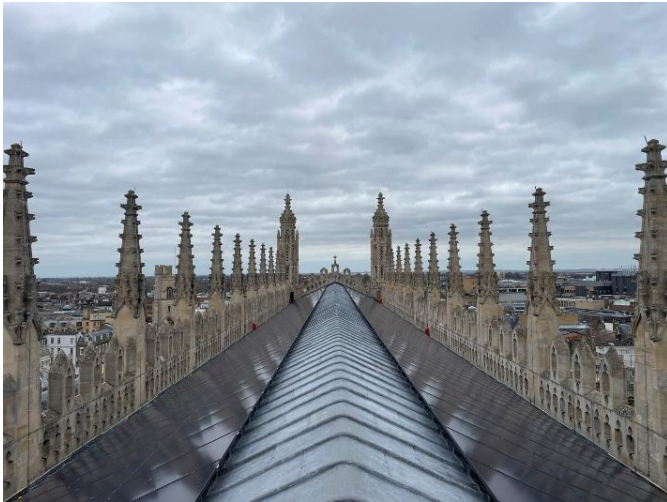
Kings College Chapel, Cambridge (all black panels, discretely visible. Mechanical fixings through lead roof)
