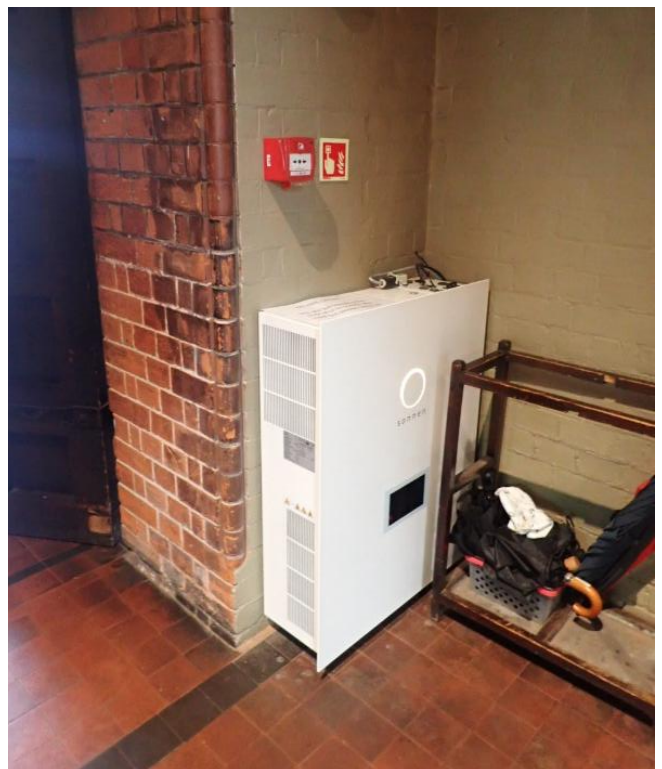
St Thomas, Finsbury Park - Combined battery and inverter
